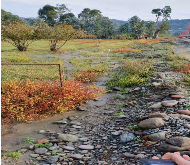
Flooded land plot owned by adjacent to stone column construction site
