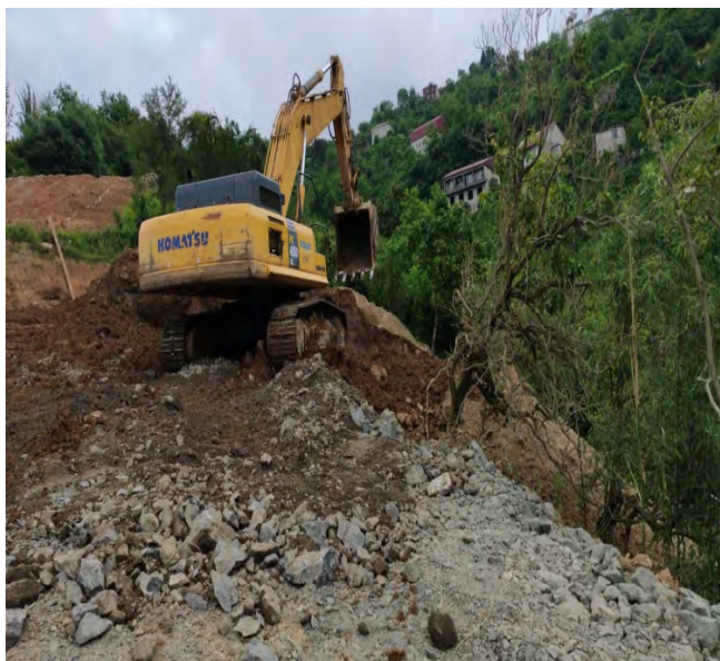
Removal of dumped soil from land plot
